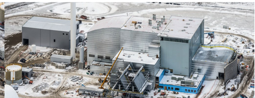
Aerial View of DYEC, looking West – January 2014
