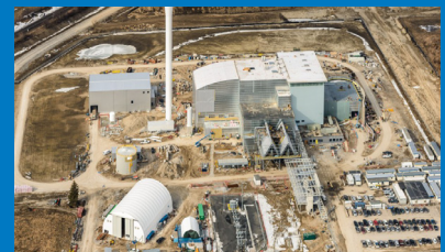
Aerial View of DYEC Construction Progress - March 2014
