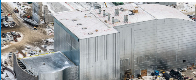
Aerial View of DYEC Construction Progress – January 2014
